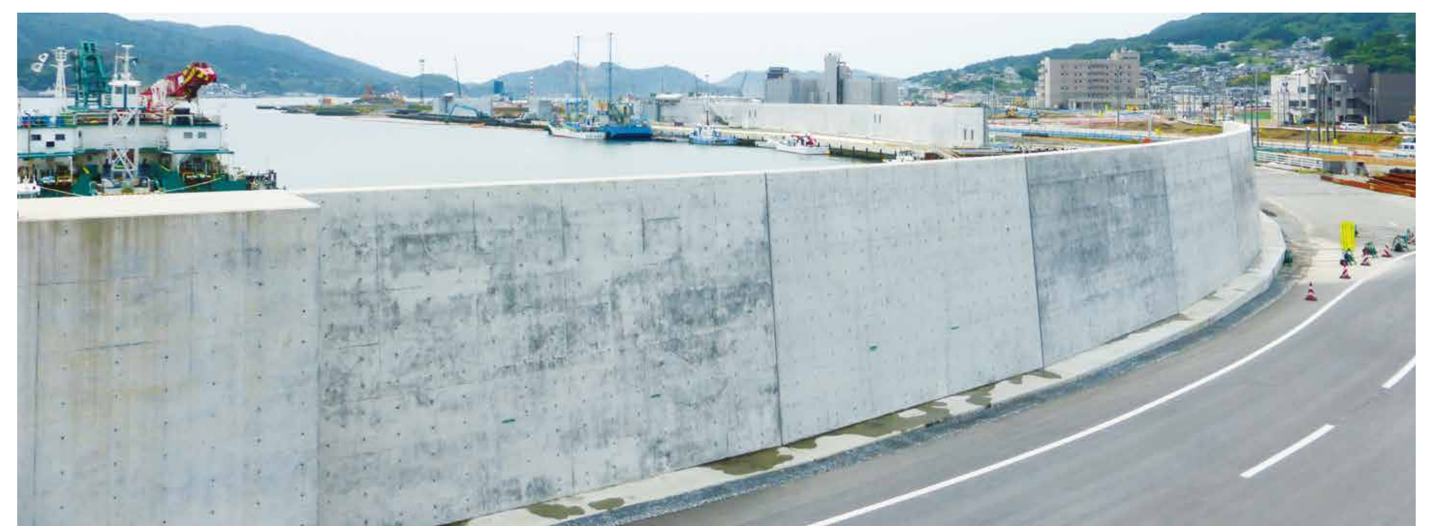
A seawall (7.5 m) in Ofunato Bay *6
